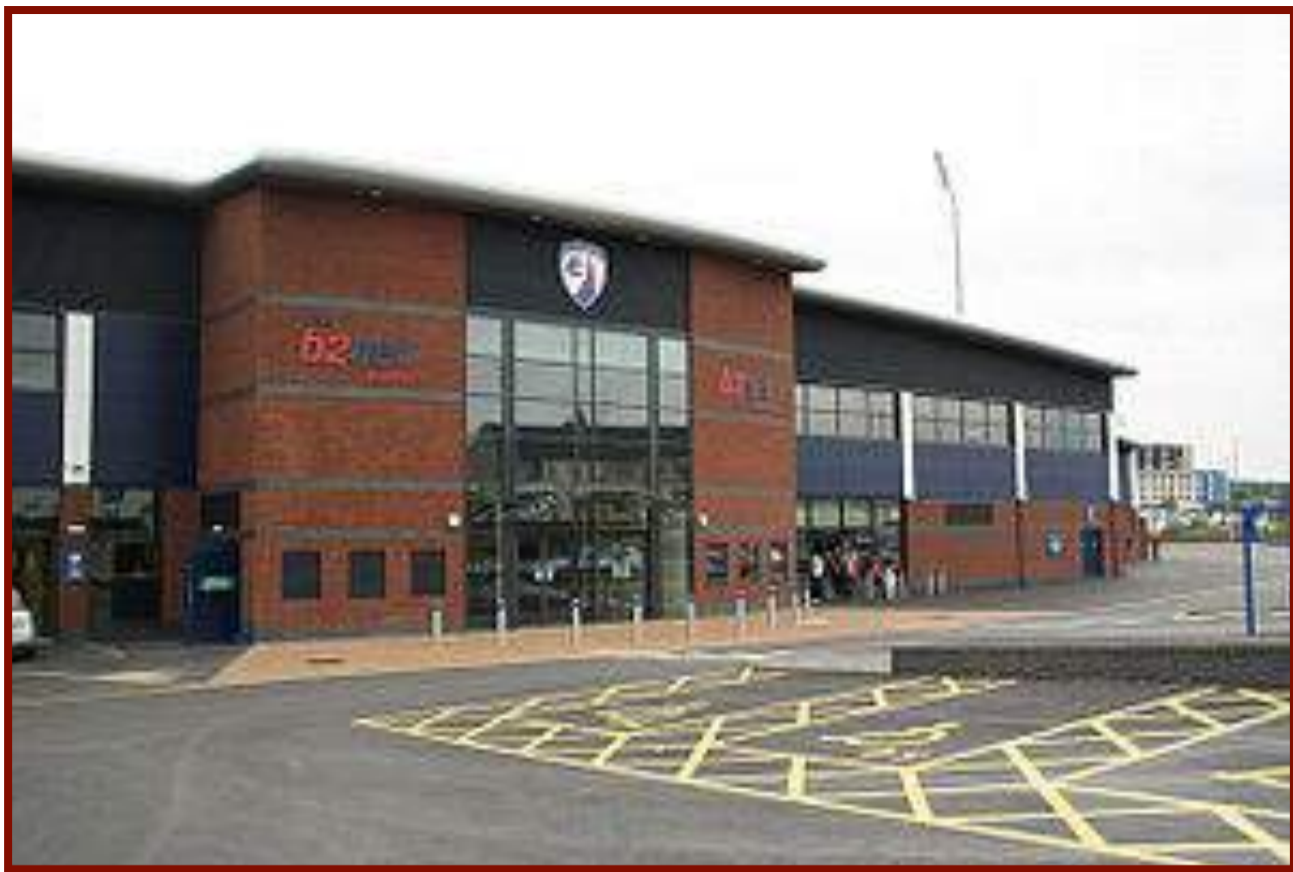
Proact Stadium, Sheffield Rd, Chesterfield S41 8NZ
